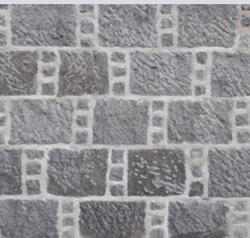
'Aberdeen Bond' – an economical use of smaller stacked blocks of granite, within the masonry courses.
