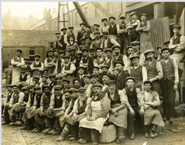
Workmen at Victoria Road Granite Works
